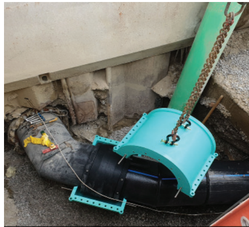
Shown above, the 114 Bell Repair design has an expanded middle section that accommodates the outside diameter and laying length of the coupling with end flanges that transition down to fit on the outside diameter of the pipe. As a mechanical joint fitting, the 114 has both sidebar gaskets and end gaskets that provide the watertight seal around the leaking coupling.
