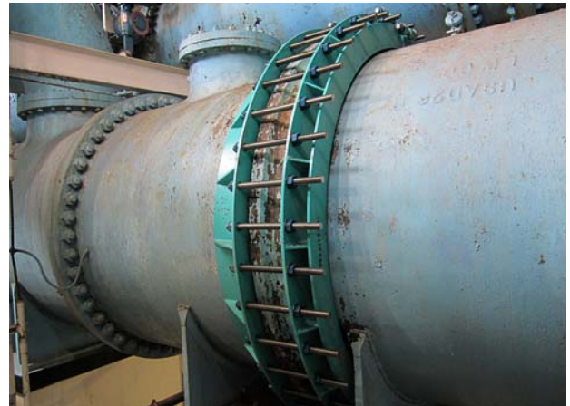
60" Treatment Plant Installation
