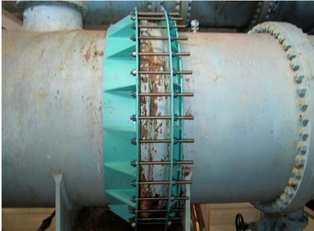
60" Treatment Plant Installation
