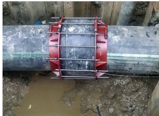
Repair of fused joint on HDPE
